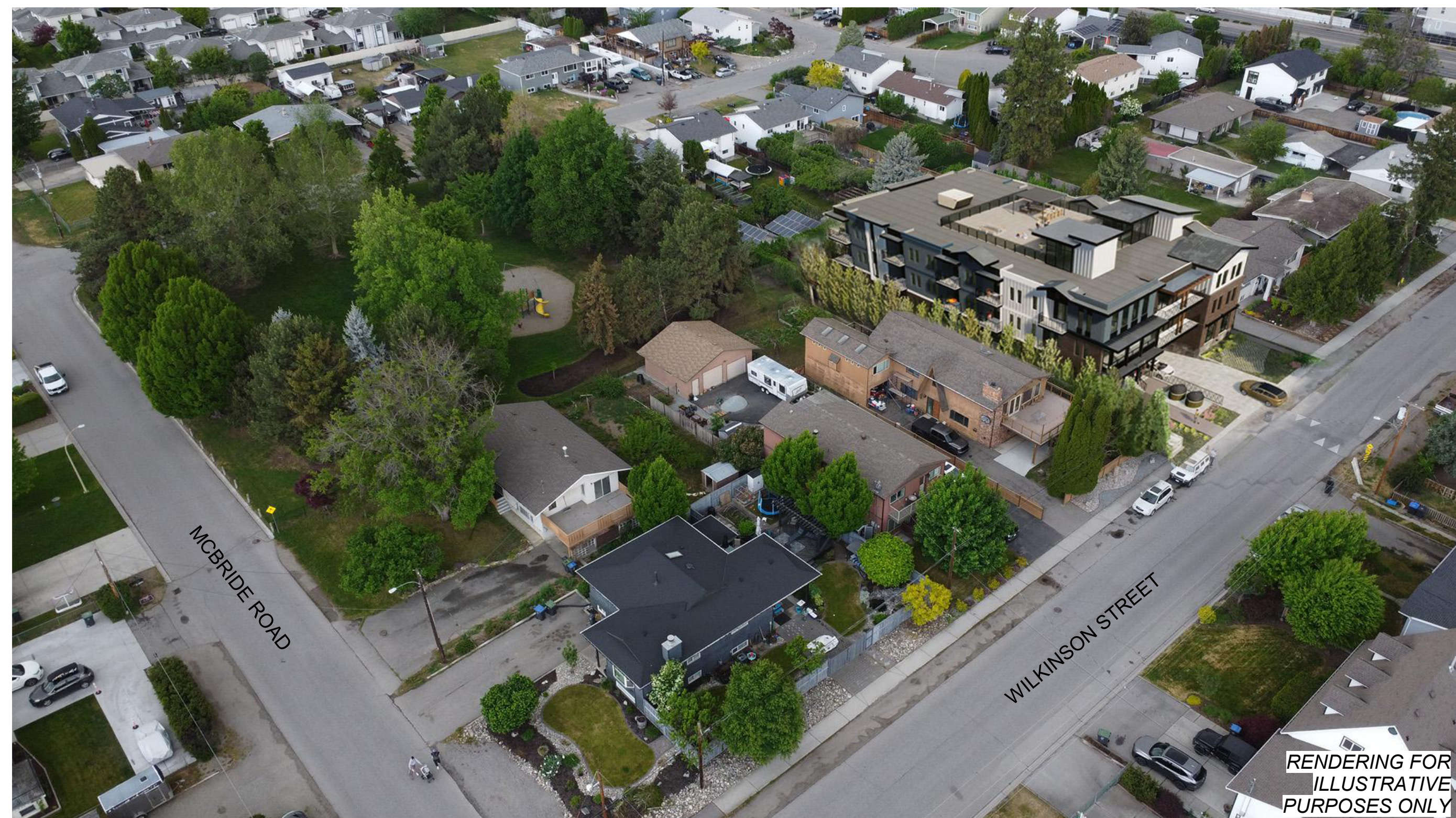
AERIAL CONTEXT VIEW FEATURING PARK
